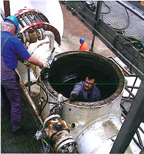
Repairing a ball valve.
