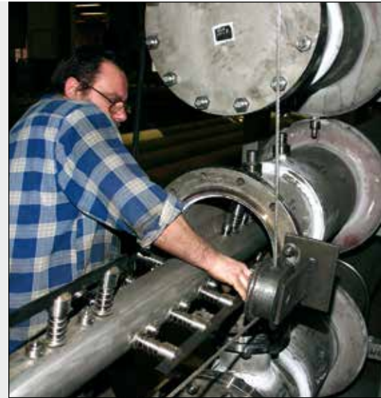
Installation of scraper shaft
