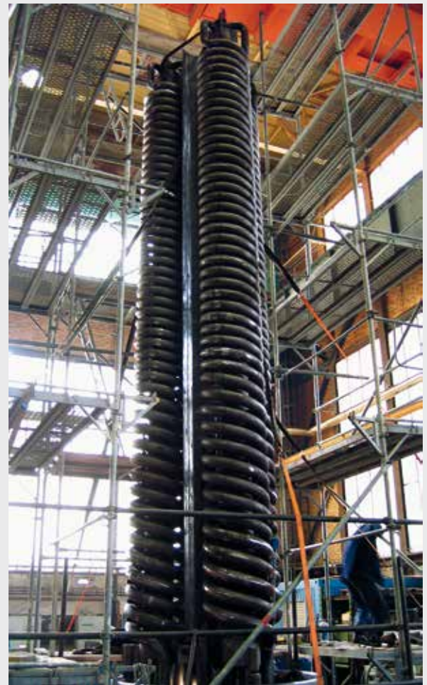
Assembly of coils
