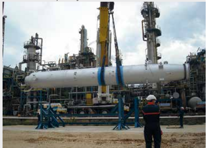
Arrival of BORSIG synthesis gas cooler at site
