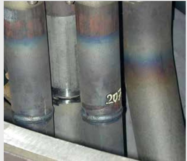
Fitting and welding of heating surfaces to connecting tubes
