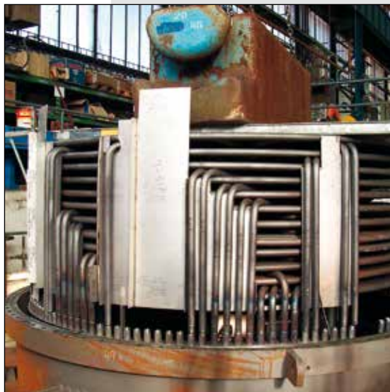
Installation of metal shroud
