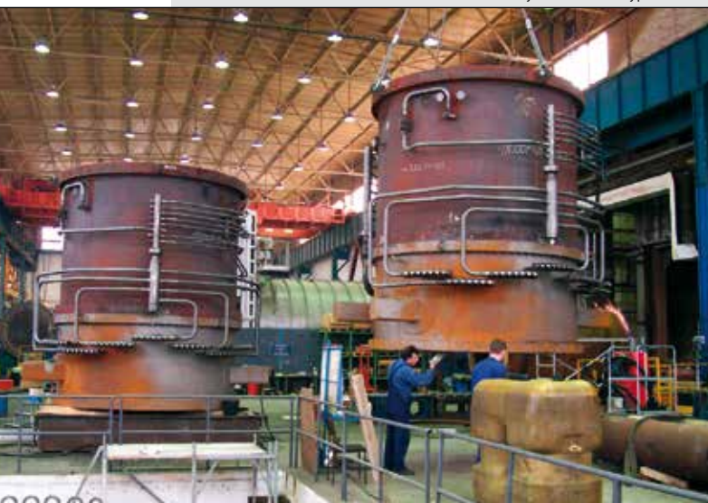
Final assembly of a LaMont type boiler
