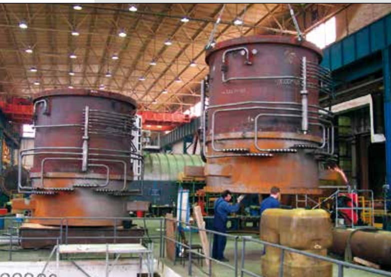
Final assembly of a LaMont type boiler
