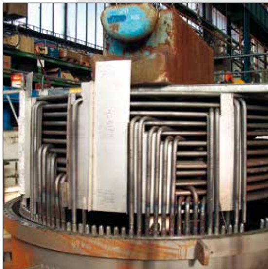
Installation of metal shroud
