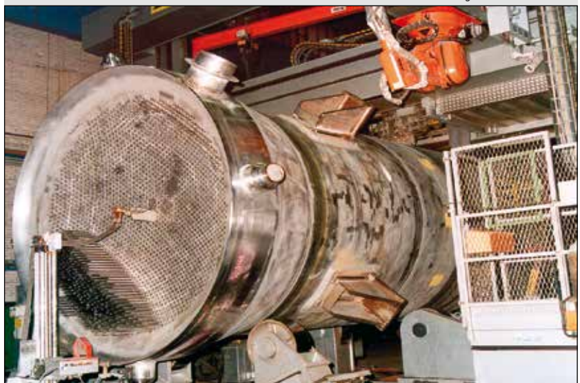
Tubesheet welding in the works area
